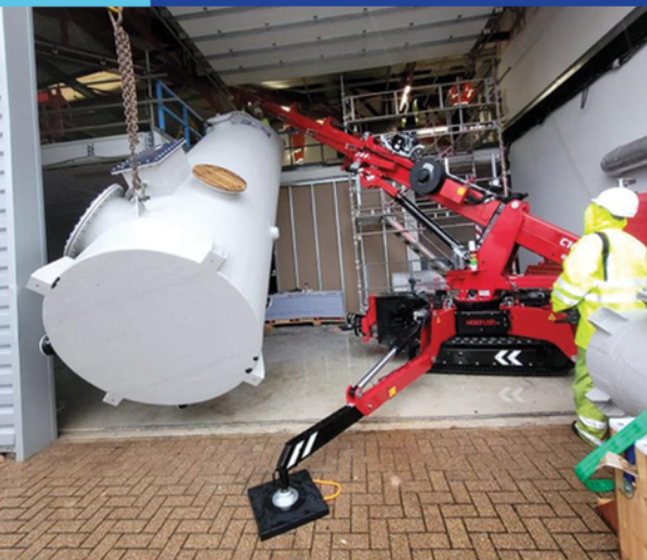
Complex installation of the scrubber into the building and tight layout of ductwork, fans, attenuator and stack in the roof-space
