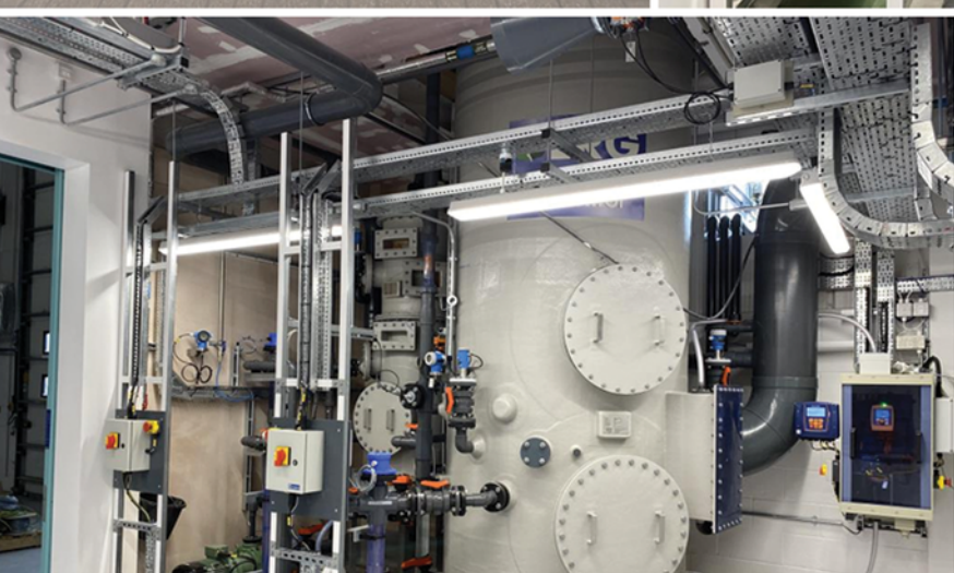
Complex installation of the scrubber into the building and tight layout of ductwork, fans, attenuator and stack in the roof-space
