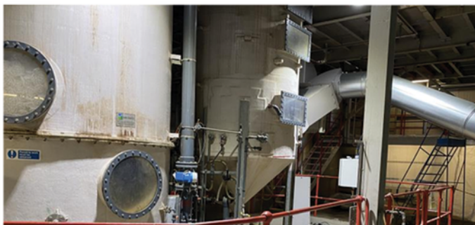
Demister and steam-fed duct heater to condition the air for carbon treatment
