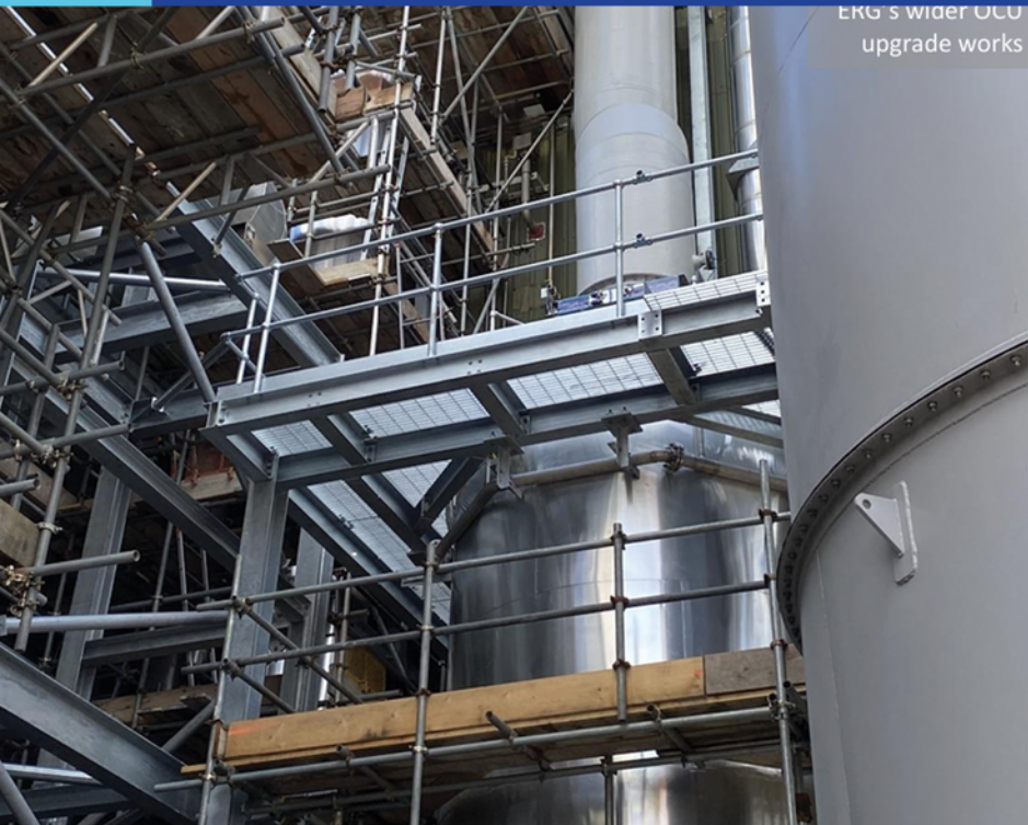
Original 1990s scrubber upper section rotated to accommodate ductwork to the heater and carbon filter, then ducted back to the original stack
