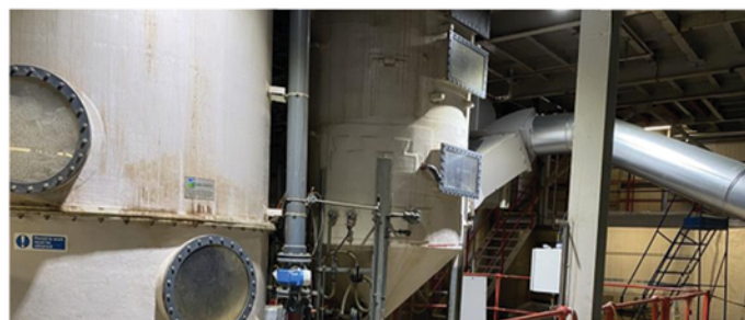
Demister and steam-fed duct heater to condition the air for carbon treatment
